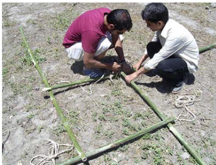
EASY KNOTTING OF JOINTS FOR POST-DISASTER SHELTER
