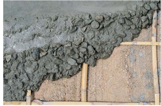
BAMBOO REINFORCEMENT IN A TEMPORARY STRUCTURE
